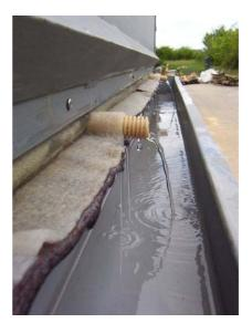
Figure 9. the flow in the draining mat is perpendicular to the mini-drains
