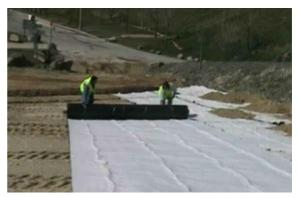
Figure 3. Installation of the geocomposite ant the top soil
