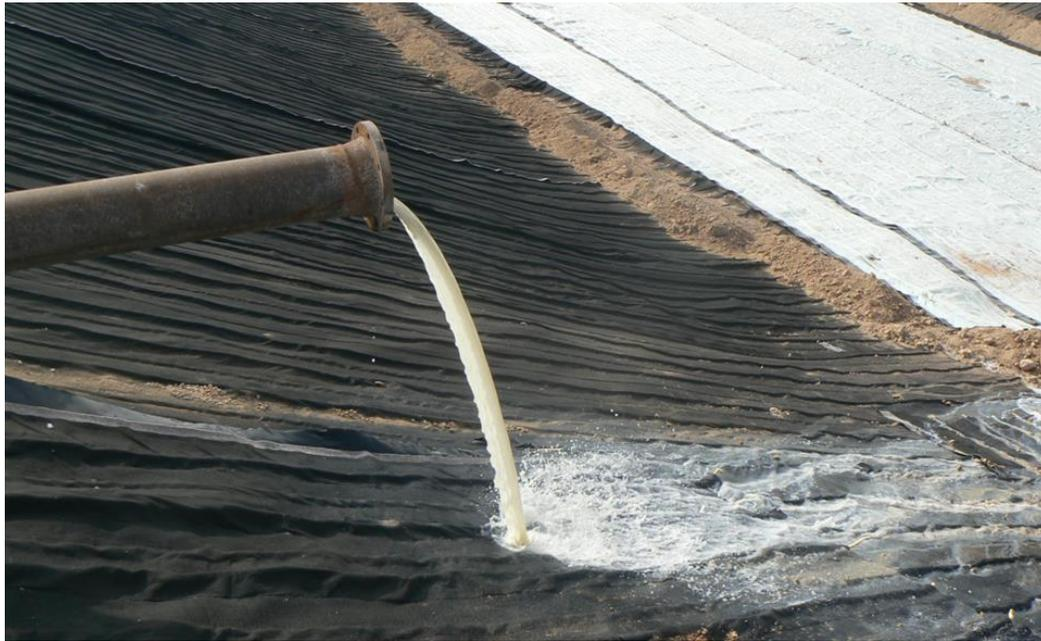
Figure 13: multi-linear drainage geocomposite used in a slurry dewatering facility (photo courtesy Afitex-
