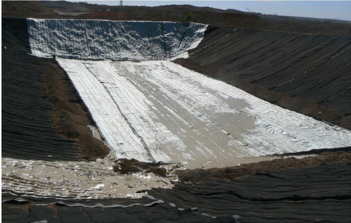
Figure 14: Slurry dewatering facility (photo courtesy Afitex-Textel)
