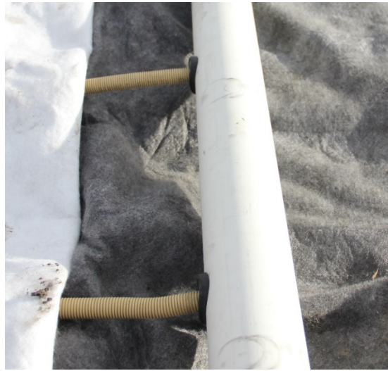
Figure 4. Connection to the collector pipe
