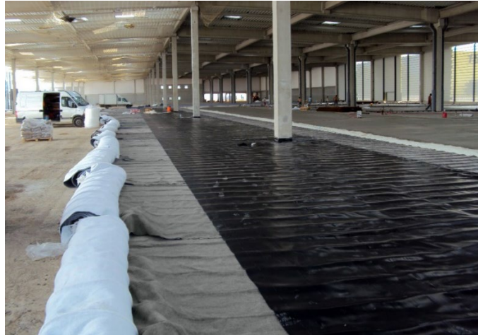
Figure 6. SSD installation under geomembrane
