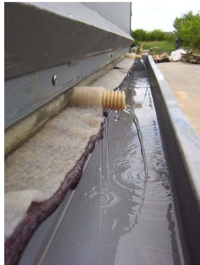
Figure 9. the flow in the draining mat is perpendicular to the mini-drains
