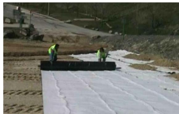
Figure 3. Installation of the geocomposite and the top soil
