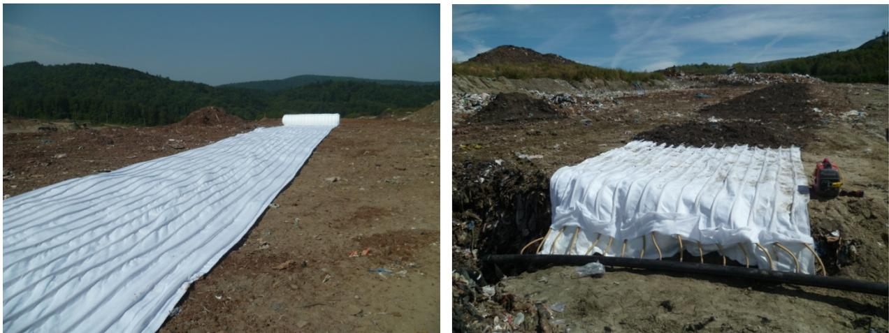
Figure 5. Tubular drainage geocomposite installation and connection to the header pipe.
