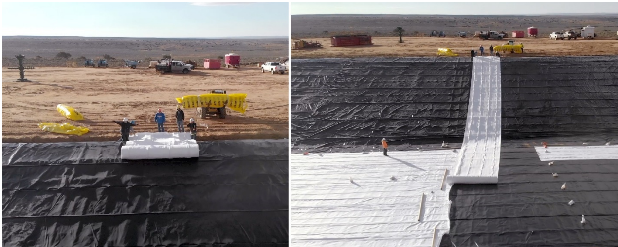
Figure 6: Deployment of the conductive multi-linear DRAINTUBE from the top of the slope
