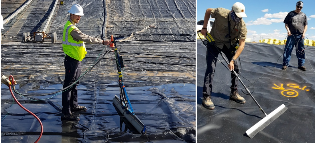
Figure 7a: Water puddle method; Figure 7b: Arc test method
