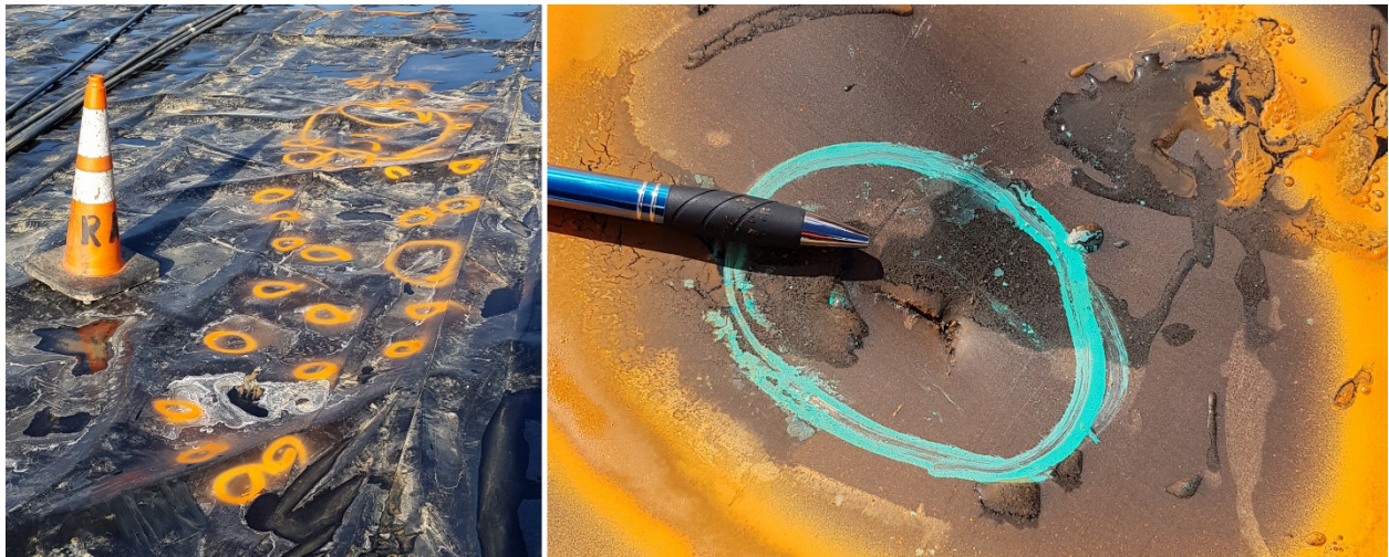
Figure 8: Example of leaks found on the primary liner at the bottom
