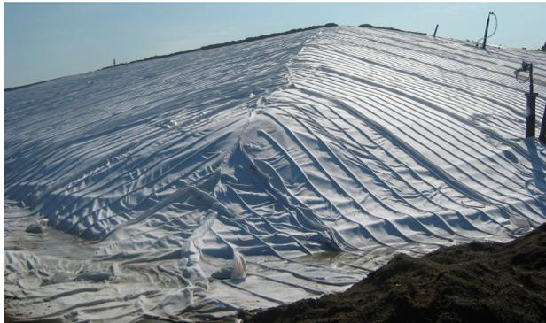
Figure 3. Exposed drainage geocomposite during installation.
