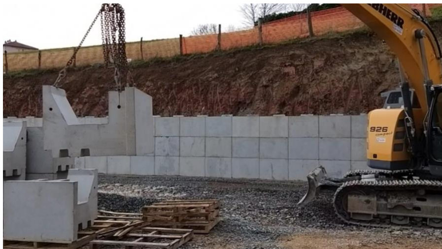
Figure 2. Illustration of the block-lifting process.
