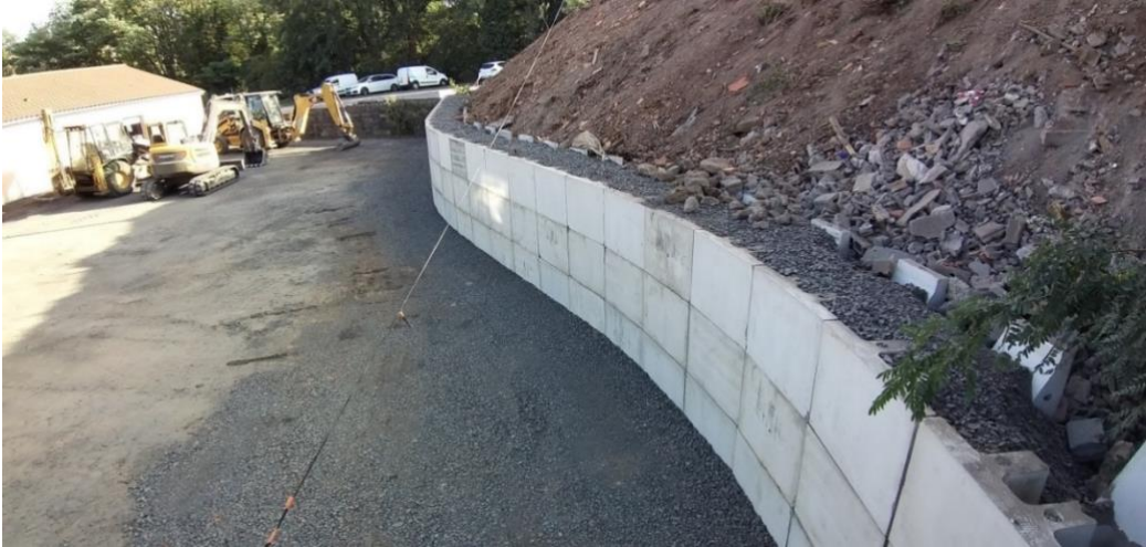
Figure 4. Test working site.
