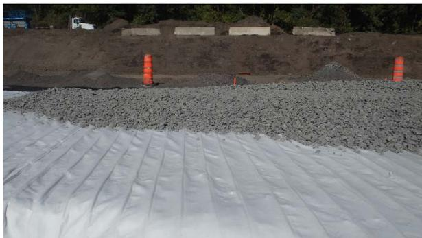
Figure 4: Putting into place of the ballast
