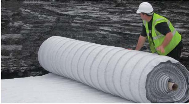
Figure 2. Roll of Draitube
