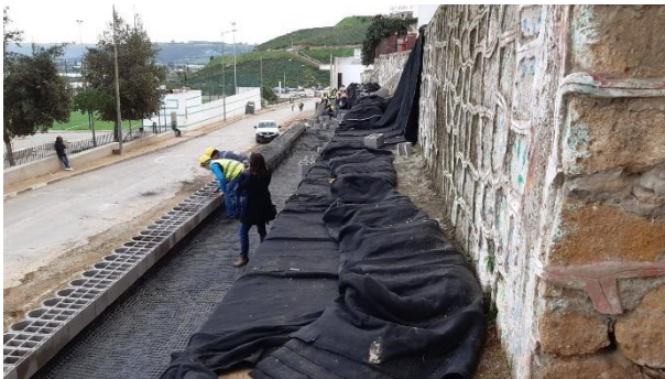
Layout of the grids, blocks and drainage geocomposite
