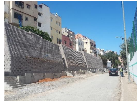
Layout of the grids, blocks and drainage geocomposite
