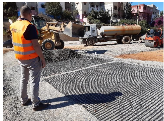
Installation damage campaign on site supervised by AFITEXINOV
