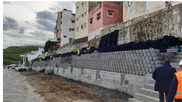
Layout of the grids, blocks and drainage geocomposite
