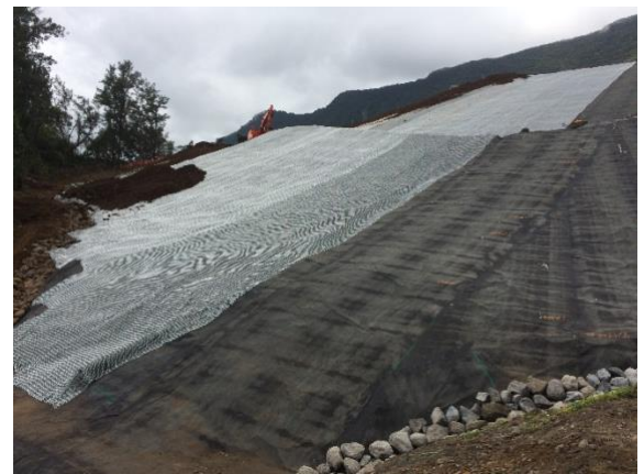
Start of AFITER 3D installation and weighting
