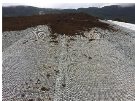
Backfilling on soil retention netting
